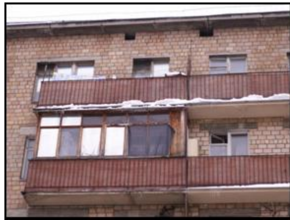
Apartment unit in a Moscow building of 1960s construction with a poorly insulated attic and open windows to release heat from the overheated radiators within.
